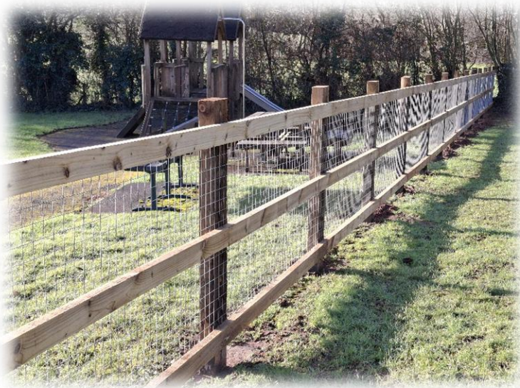
New fencing around the Children's Play Park area
