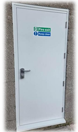
One of the new Fire Doors at the Pike Den
